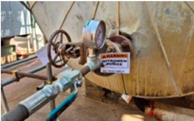
Nitrogen purging of static equipment in progress
