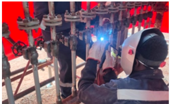
Piping Work in progress
