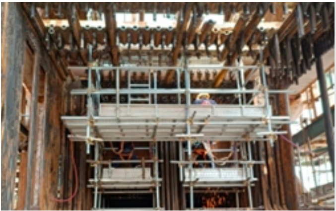
Boiler tube revamp in progress
