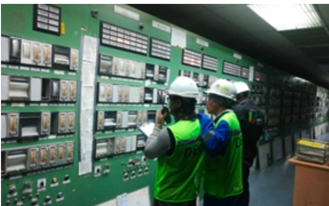
Loop test of control room in progress
