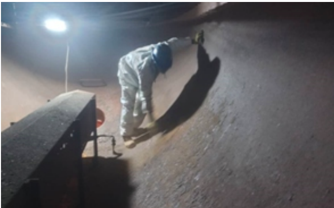
Internal Cleaning of Drums
