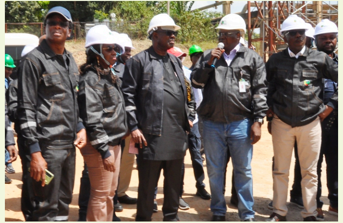
The MD, KRPC, Dr. Mustafa Sugungun (2nd right) explaining the level of progress of the project to the HMSPR, Oil, Sen. Heineken Lokpobiri ; GCEO, NNPC Limited, Mele Kyari (1st right); Executive Vice President, Upstream, Oritsemeyiwa Eyesan (second left); Executive Vice President, Downstream, Adedapo Segun (first left)
