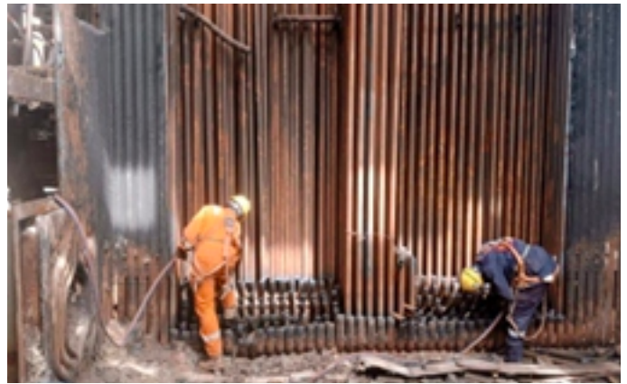
Boiler-1 main bank tube cutting in progress
