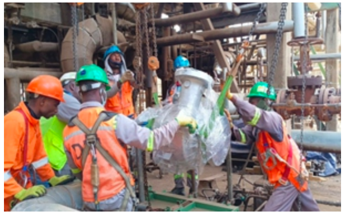
Overhauled pump re-installation
