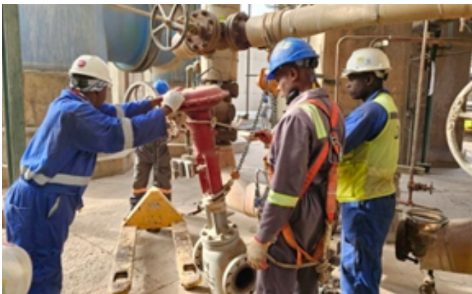
Control Valve Removal
