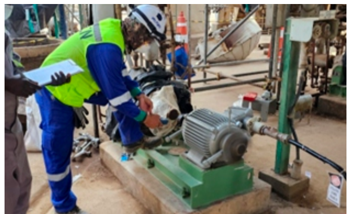
Motor solo run test in progress
