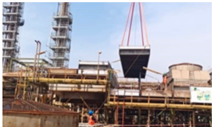
Air Fin Fan Cooler - Tube Bundle revamp in progress
