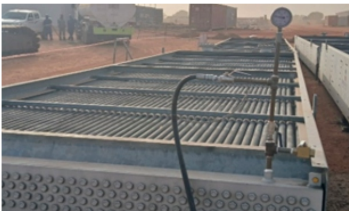
Air Cooler Tube Bundles Air-blowing & Hydrotest in progress
