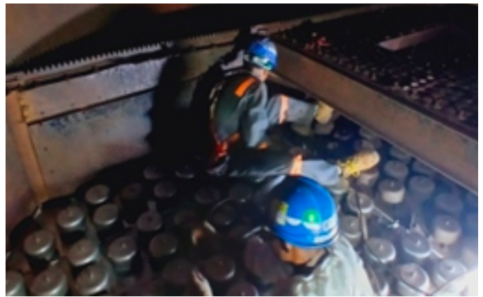
Crude Distillation Unit 1 internal tray revamp in progress
