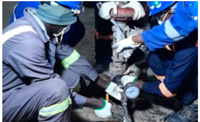
Control valve leak test in progress
