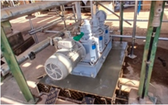
Pump Foundation completed
