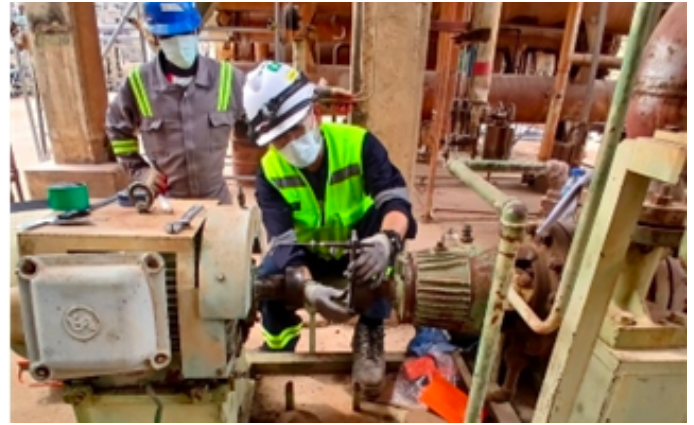
Area 1 work alignment in progress
