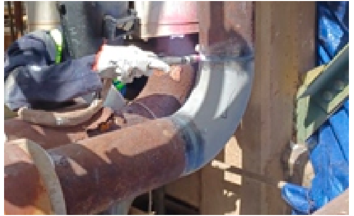
Piping Replacement Work
