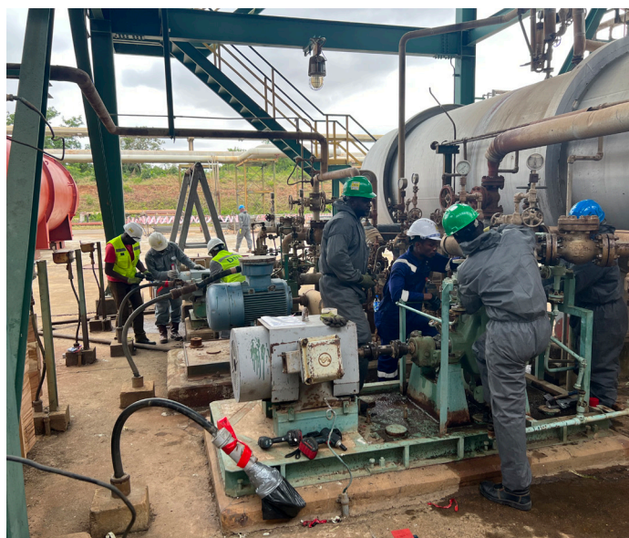
DECN crew dismantling pumps for overhaul
