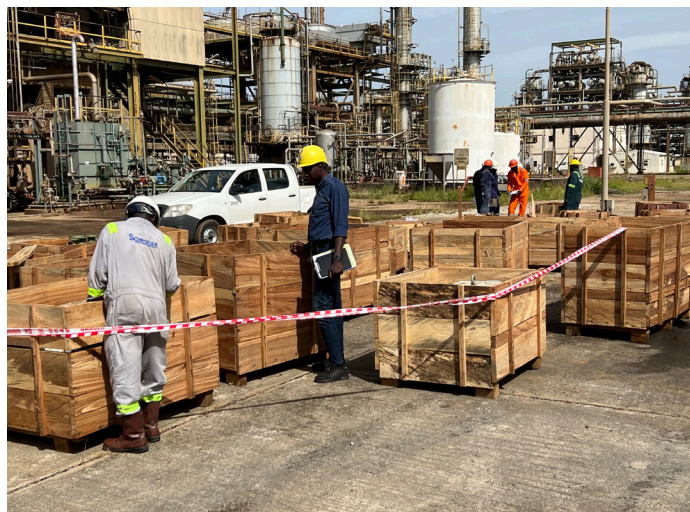
First batch of dismantled pumps ready for movement to BEAMCO for overhaul
