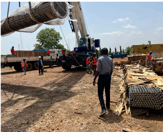
KRPC and Daewoo Project Team supervising delivery of new Heat Exchanger Bundles to site
