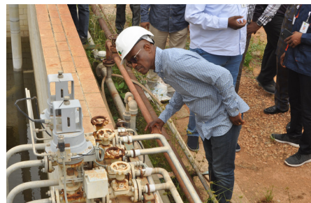
The EVP, Downstream Engr. Adeyemi Adetunji inspecting the Waste Water Treatment Plant
