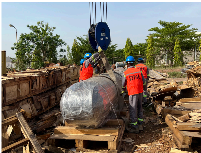
New Heat Exchanger Bundles from KRPC warehouse being delivered to site
