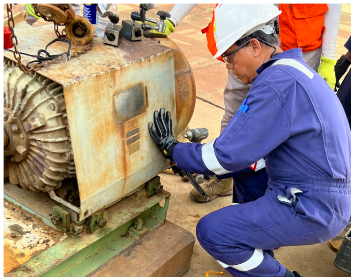
BEAMCO Engineer working on one of the pumps
