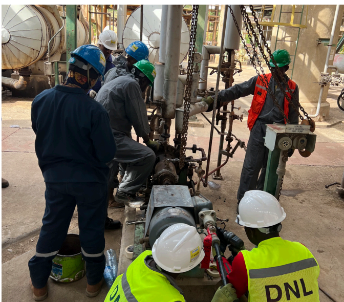
DECN Maintenance crew dismantling pumps for revamp
