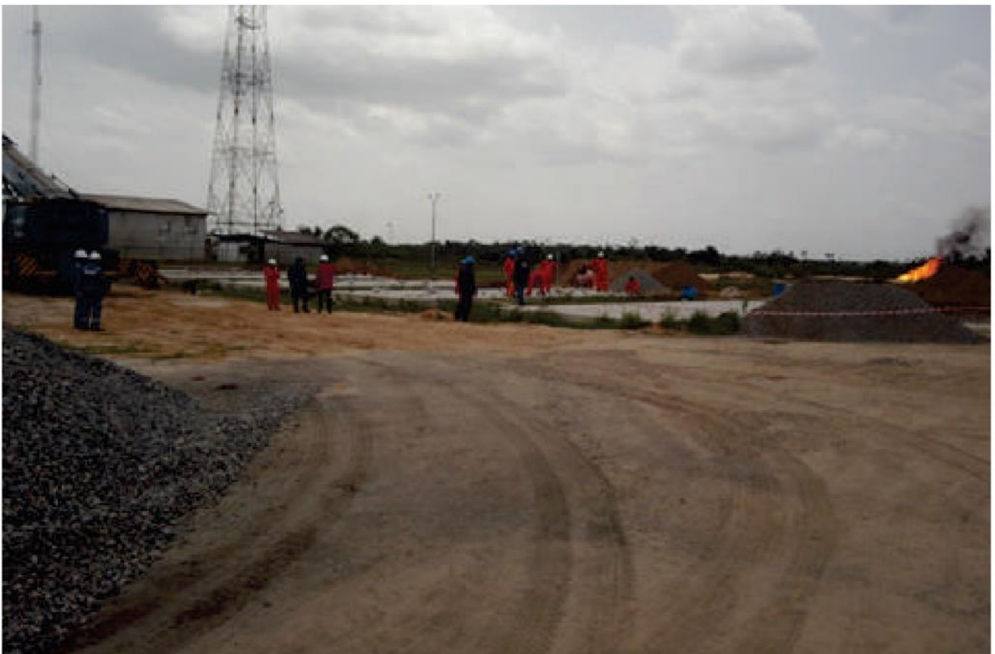
Sapele Gas Plant under construction (complete upgrade)
