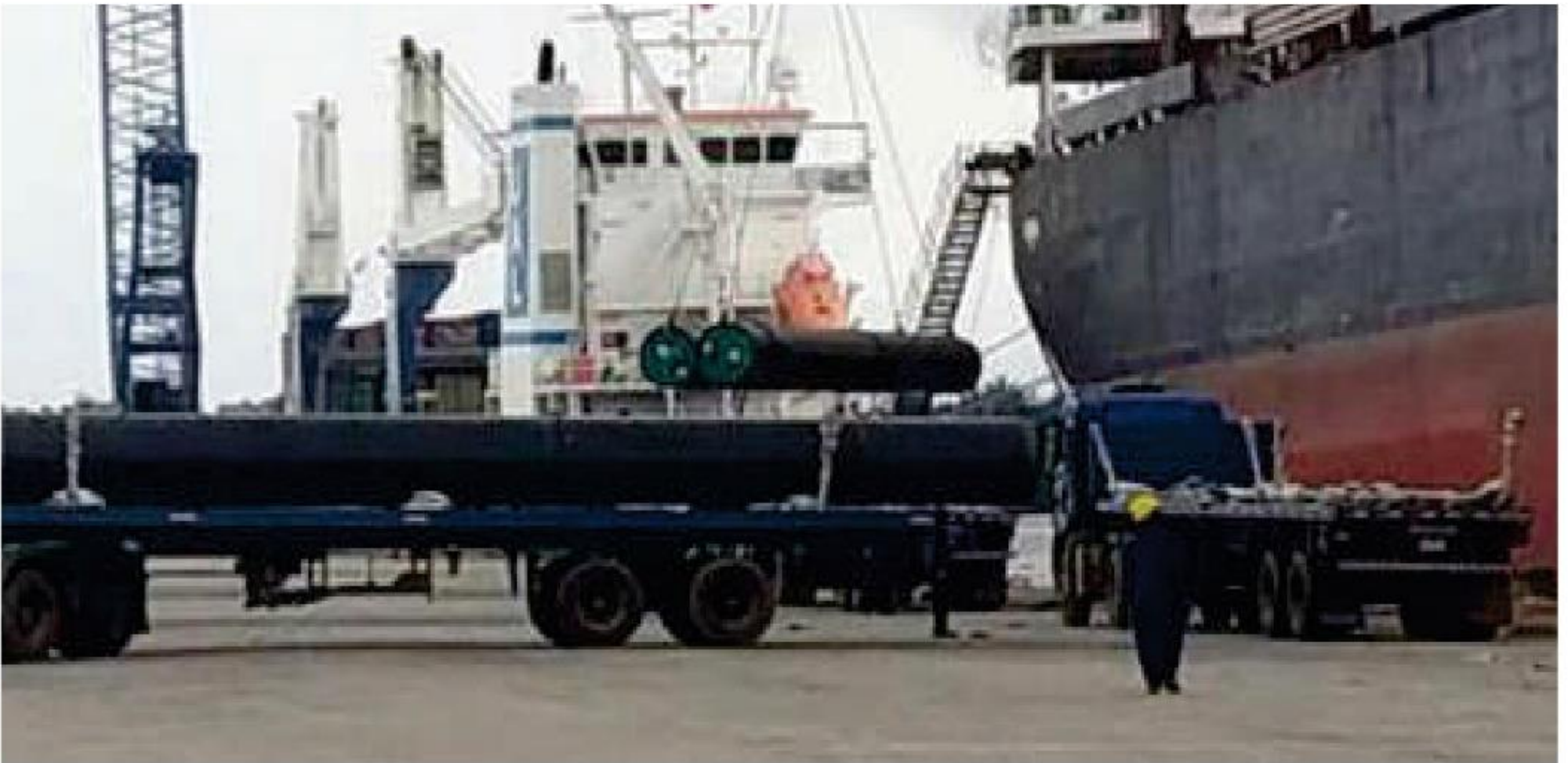
Offloading of Project Line Pipes
