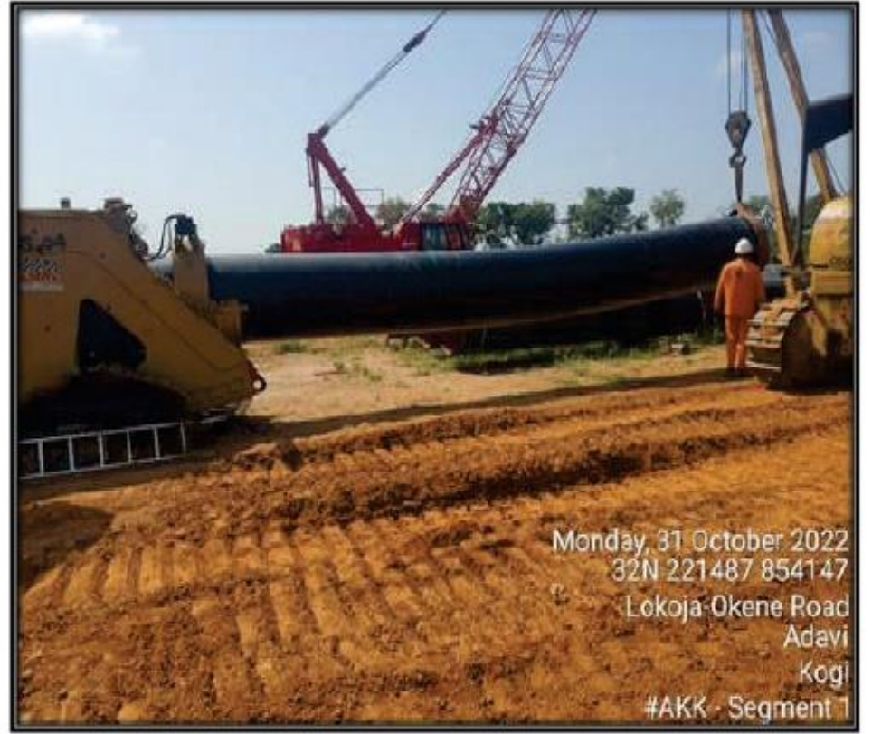
Cold Bending in progress
