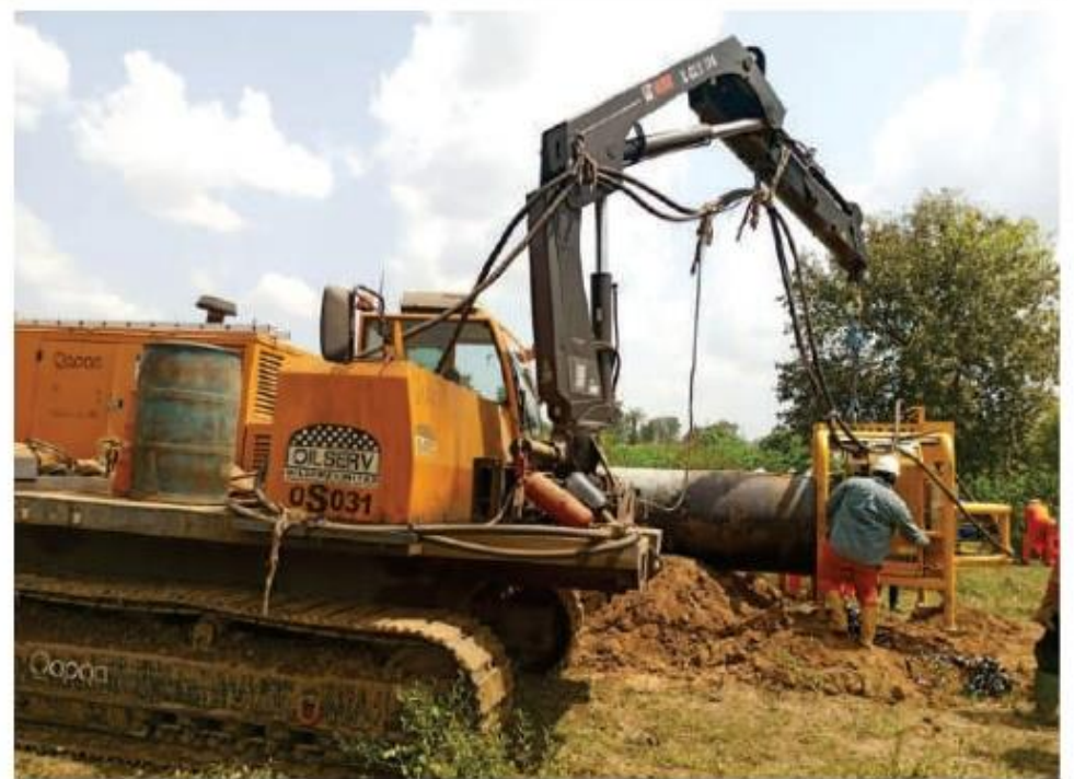
Automatic Welding Machine in action
