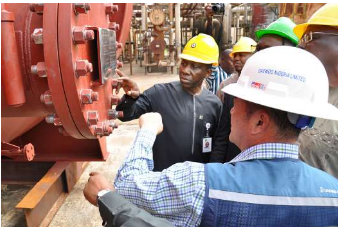
Daewoo Nigeria Limited personnel explaining the use of one of the equipment to MD NETCO and his team during the site visit to the KRPC Rehabilitation project
