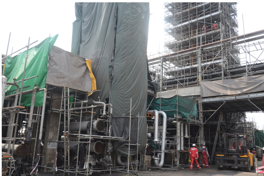
Ongoing works at Area 5
